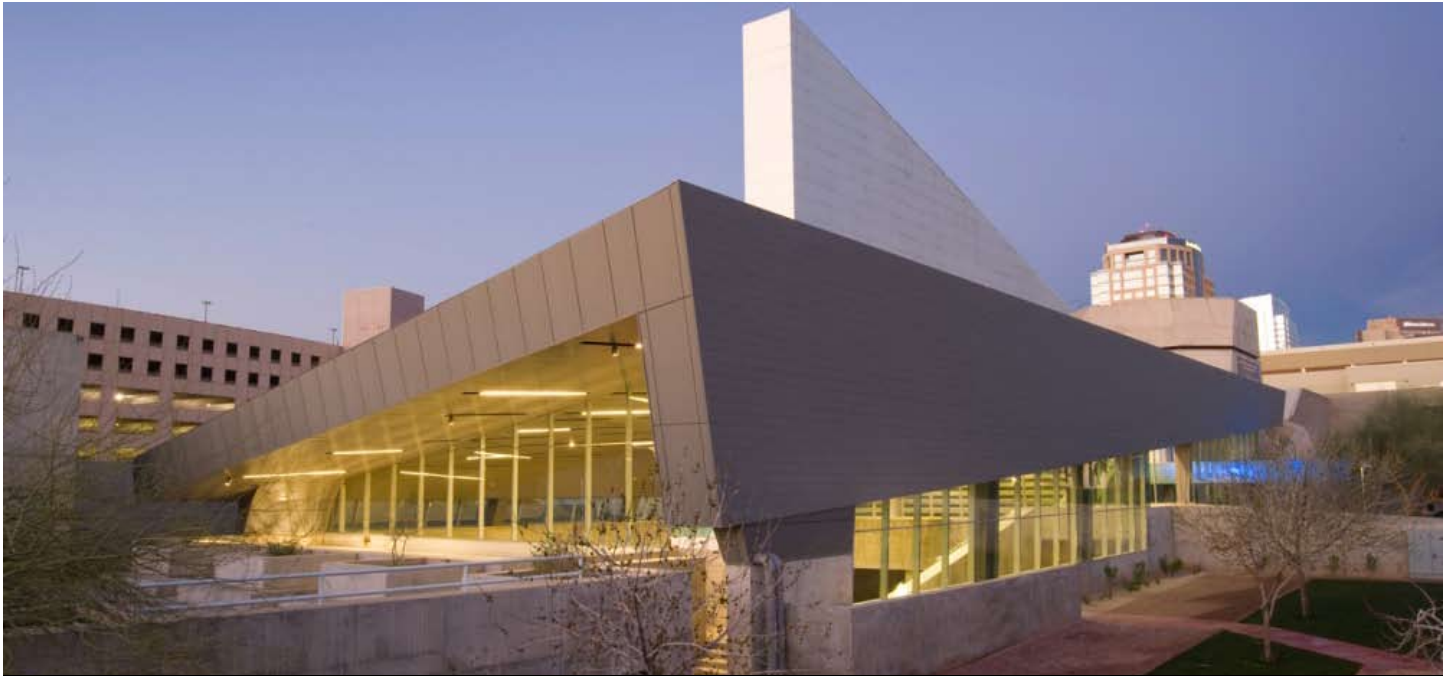
Arizona Science Center – Phoenix, Arizona Fabrication and Installation by Elward Systems Corporation
