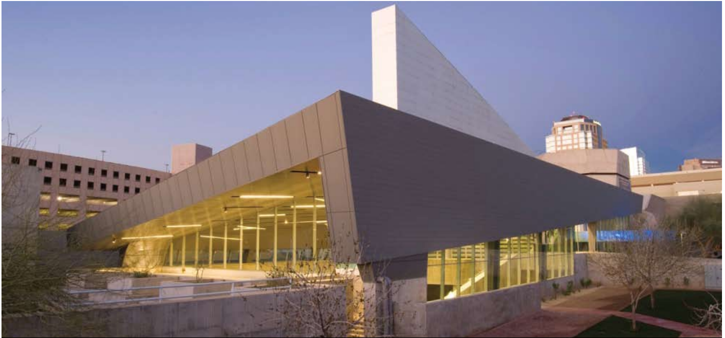
Arizona Science Center – Phoenix, Arizona Fabrication and Installation by Elward Systems Corporation
